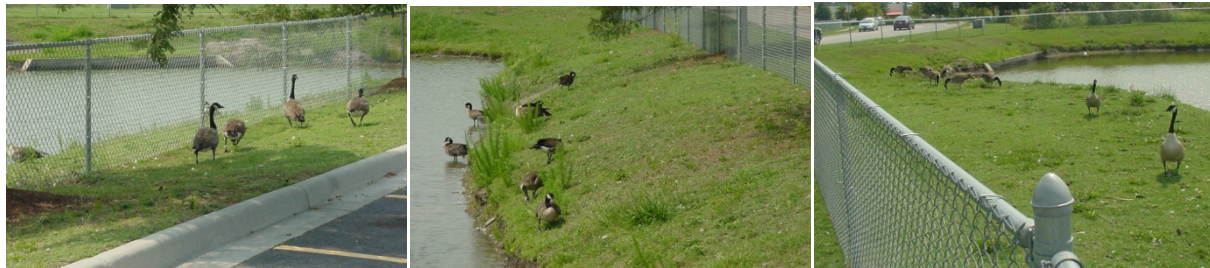
Fencing located too far from the water's edge
