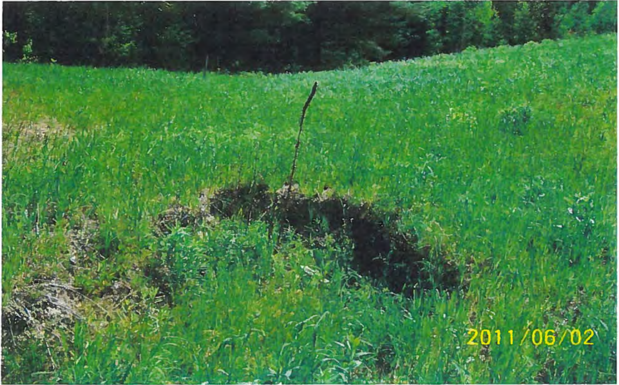
Erosion on Waste Mound
