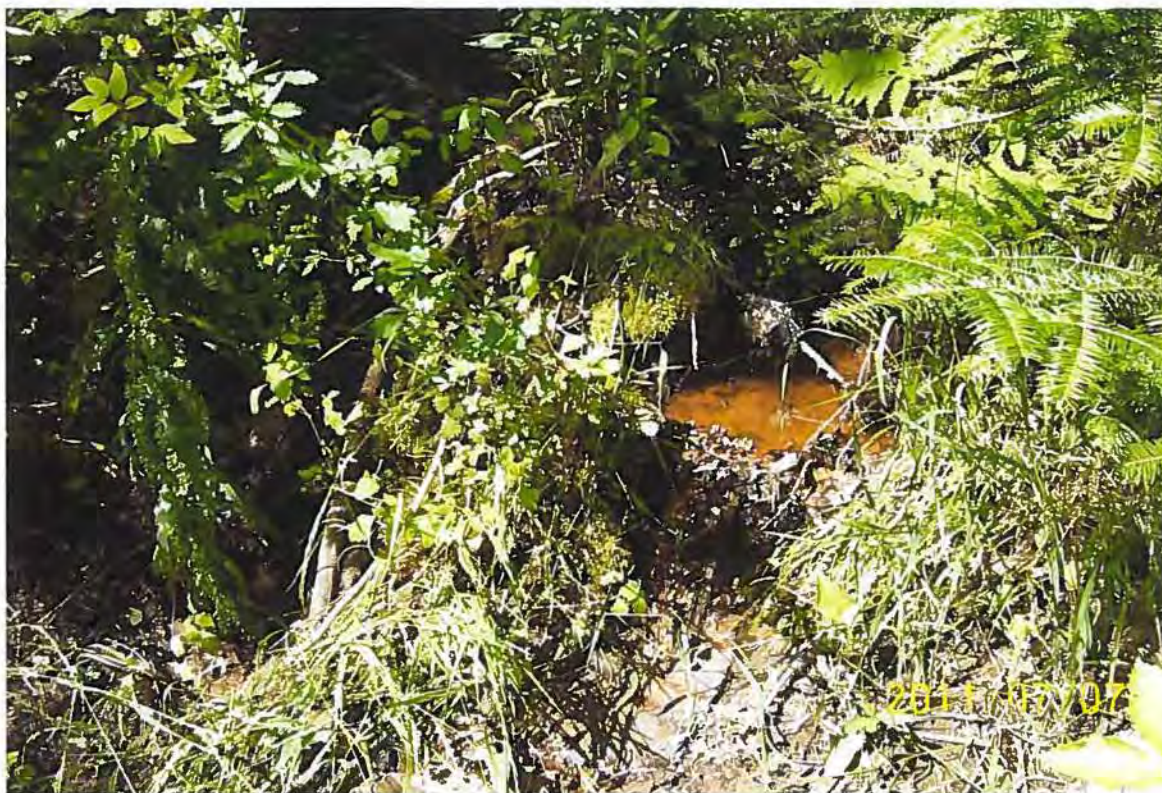
Seep 1 Location (Not Flowing)
